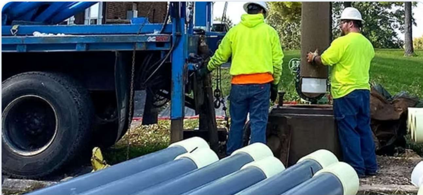
FIELD INSTALL THROUGH WATER WELL SOLUTIONS
