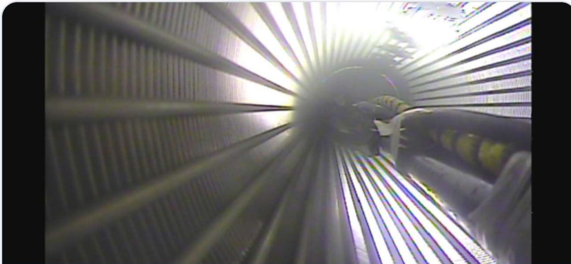
INSIDE A LATERAL SCREEN • BALLARD MARINE CONSTRUCTION
