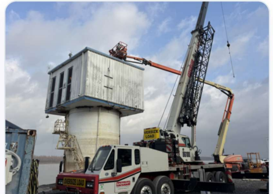
COLLECTOR-WELL CAISSON INSTALL
